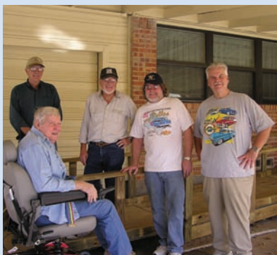
Members of Dallas Area Classic Chevys posing with the beneficiary of one of their Christmas handicap ramp building projects.
